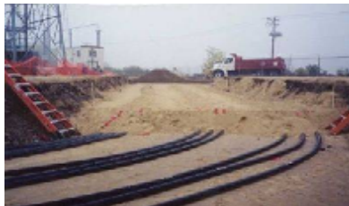
Figure 11: Installation of 400 kV XLPE cables
