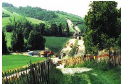
Figure 10 : cable route at site
