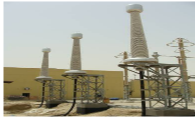
Figure 6: 400 kV Termination
