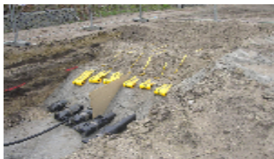
Figure 3 : 220 kV cable system pulled in pipes and buried
